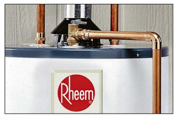
Use a new ¾ inch N.P.T drain valve
