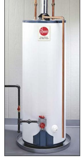
9. Turn the power ON to the water heater at the circuit breaker (electric heater) or main gas line (gas heater; relight pilot if required). Allow the water heater to recover. Check the temperature and pressure relief valve one more time to make sure it is tight.
